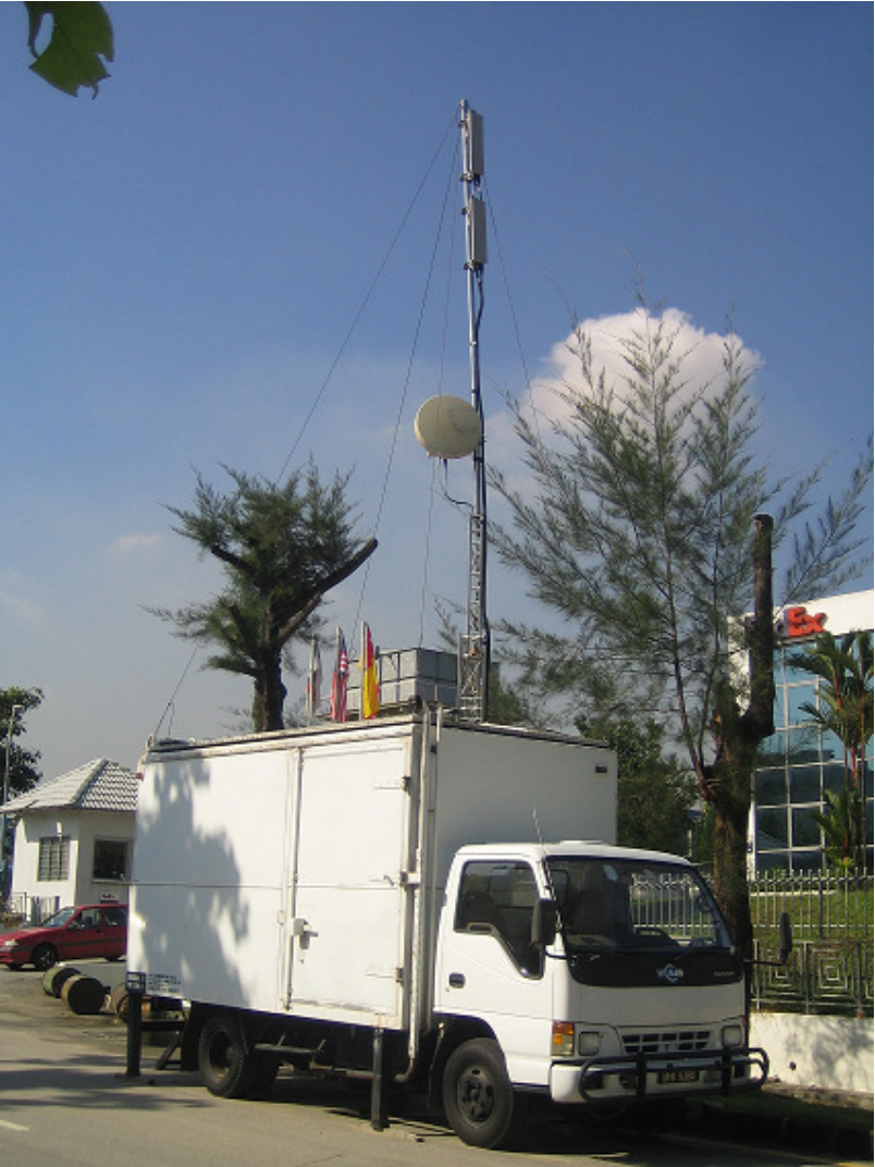
Photo 2: GSM MBTS at Subang Hi-Tech
